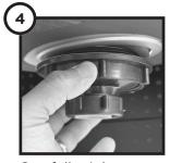
Carefully tighten basket strainer nuts in place
