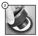
Once strainer washers are firmly in place, insert basket strainers into sink holes
