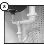
Finally, connect PVC continue waste to PVC P-trap. Carefully connect P-Trap to Wall Adapter
